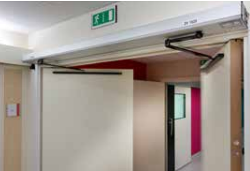
Slim, 70 mm operator for doors up to 250 kg
